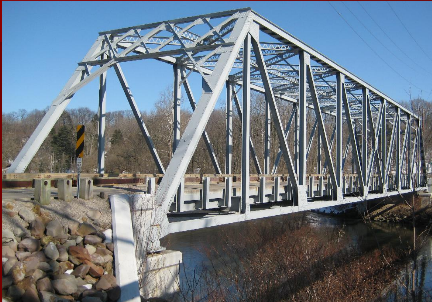
CUY Hillside Road over Cuyahoga River
